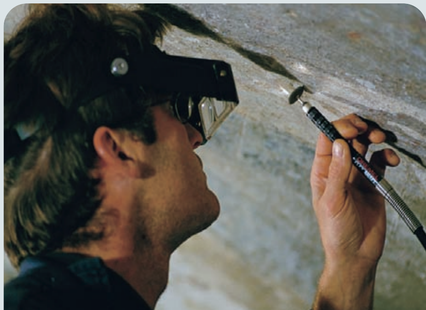
Conservation work on the Abbey.
